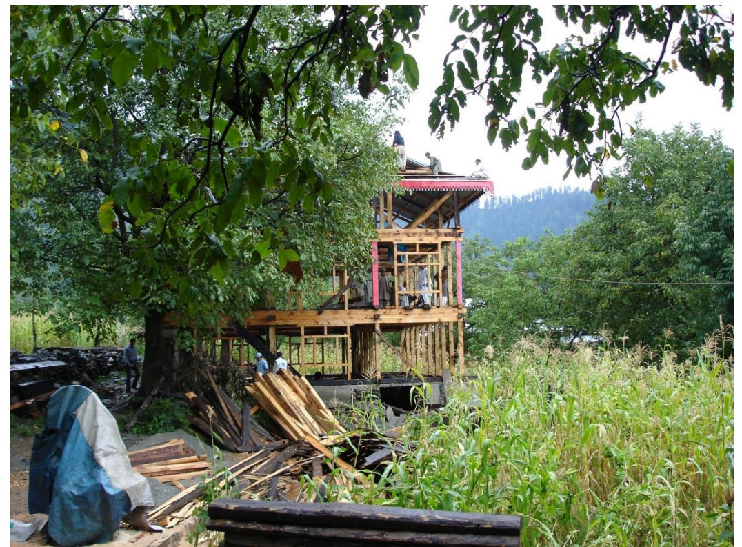
NOKOT: House of Rashid being reconstructed as a traditional house using salvaged material.
