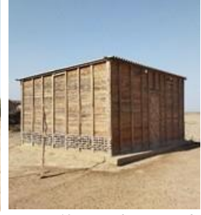
Fig 48: Warehouse made with marine ply and wood. Source: Captured by Author
