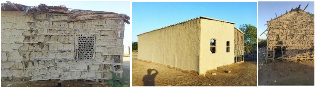
Fig 40-41-42: Different types of mud cladding techniques used by the habitants for insulation. Source: Captured by Author
