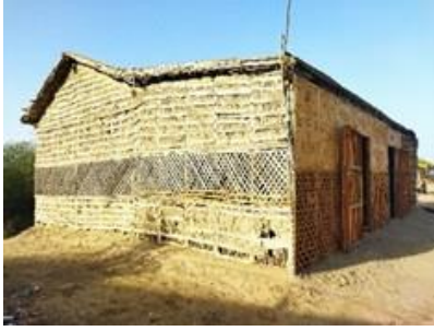
Fig 46: Walls made up of Diyar wood and mud plaster.
