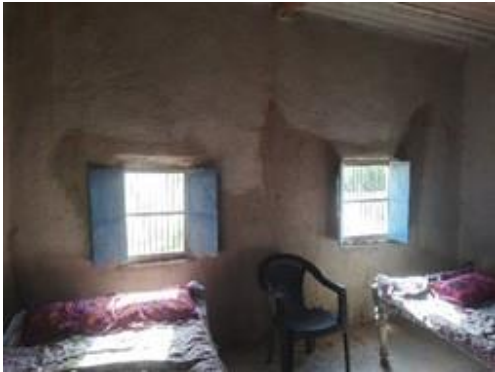
Fig 54 Placement of windows in the direction of the winds to resist heat in the house
