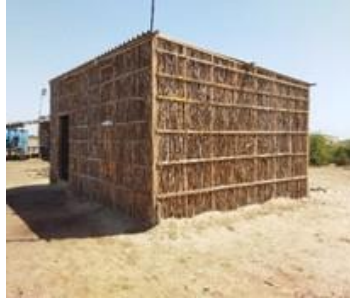
Fig 47: Shop walls built with straw bales and wood.
