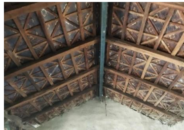
Fig 44: Roof made from marine ply and wooden logs.
