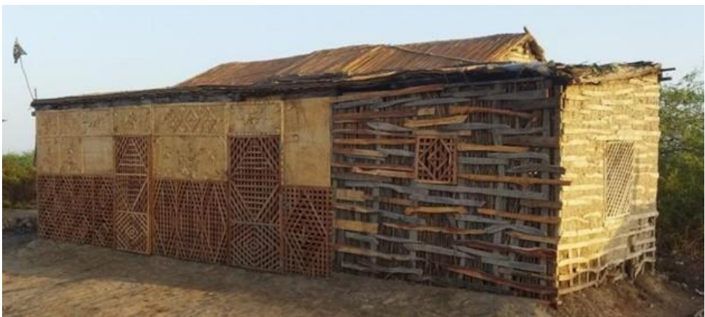
Fig 3: Shows rich indigenous construction techniques and vernacular architecture of Kharochan. Source: Captured by Author
