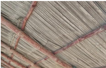
Fig 43: A thatched roof with bamboo support.
