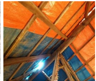
Fig 45: Wooden log roof with plastic sheet insulation. Source: Captured by Author
